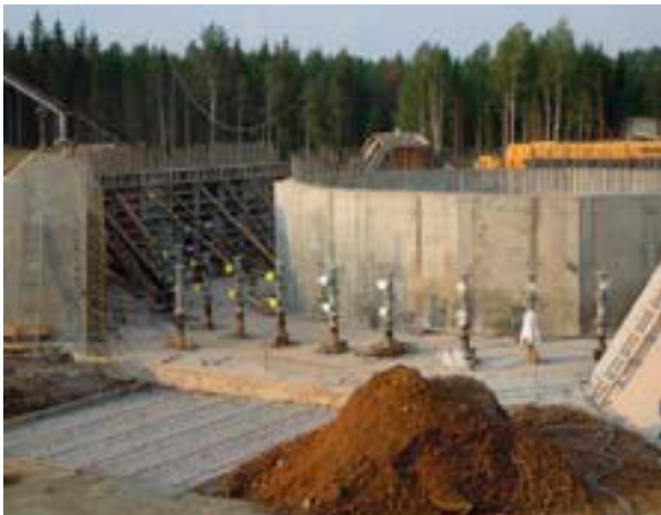
View of the construction site
